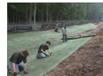
AmeriCorps members working on a drainage swale at Emerson Park.
