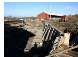
A manure storage pit under construction.
