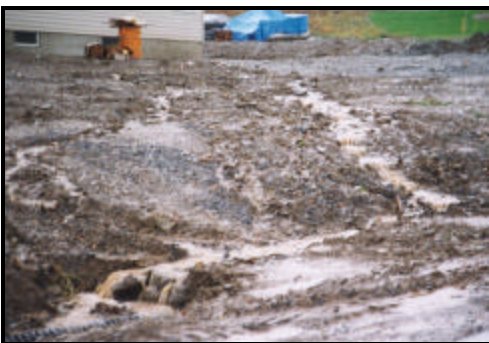
Stormwater runoff from new home development.
