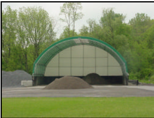
Town of Moravia salt storage shed.
