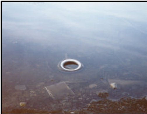
Trash dumped in Owasco Lake.
